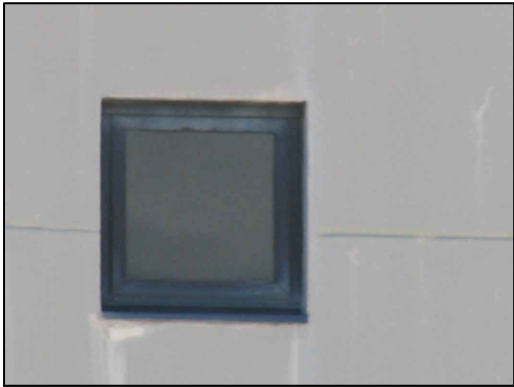
PHOTO I STREAKS AROUND WINDOW
